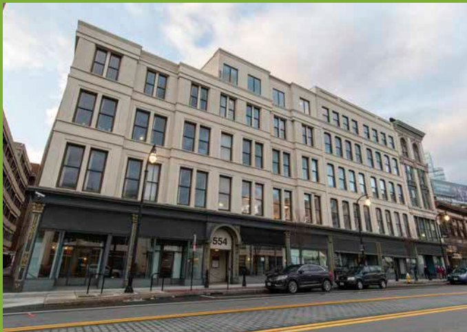
554 Main St. in the Theatre District
